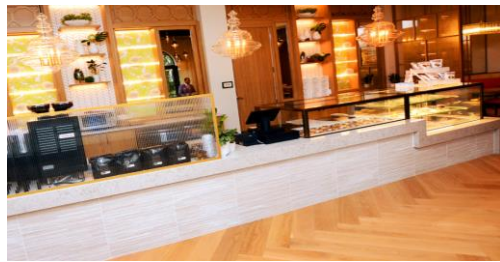
Oscartek custom cases and counters as an integral part of the remodel
